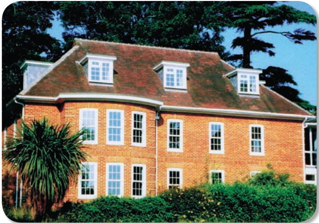
Major refurbishment of office premises
